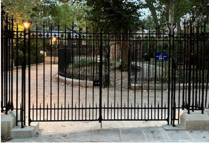
The completed gates, October 2025
